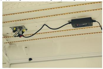
9. Install the 4 LED strips segments and connect the 4 leads.
